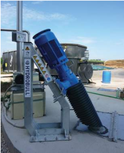
Picture: Streisal Maischebull® / Hydrobull® agitator system for mixing pits and hydrolysis tanks
