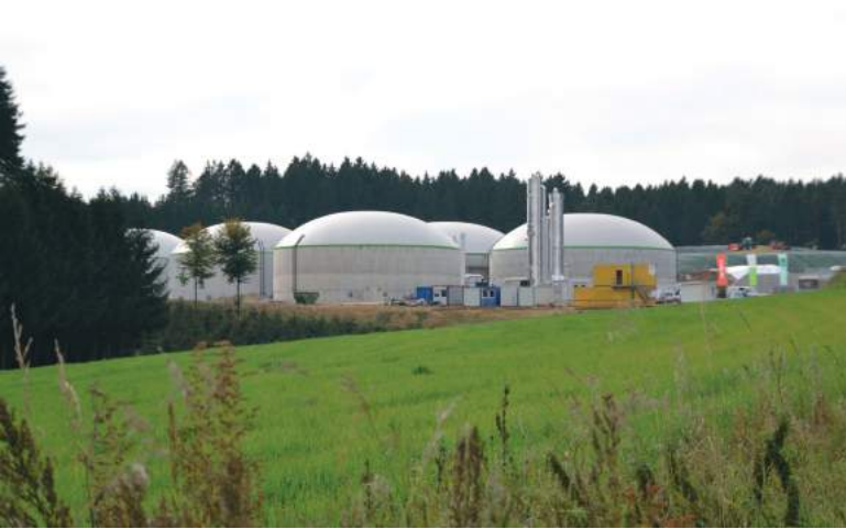
Picture: Oberlauterbach plant Schmack Biogas GmbH
