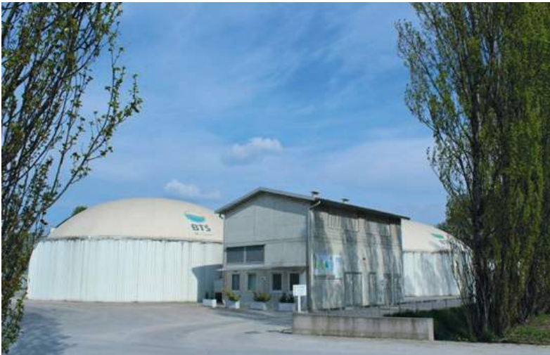
Picture : BTS Biogas
