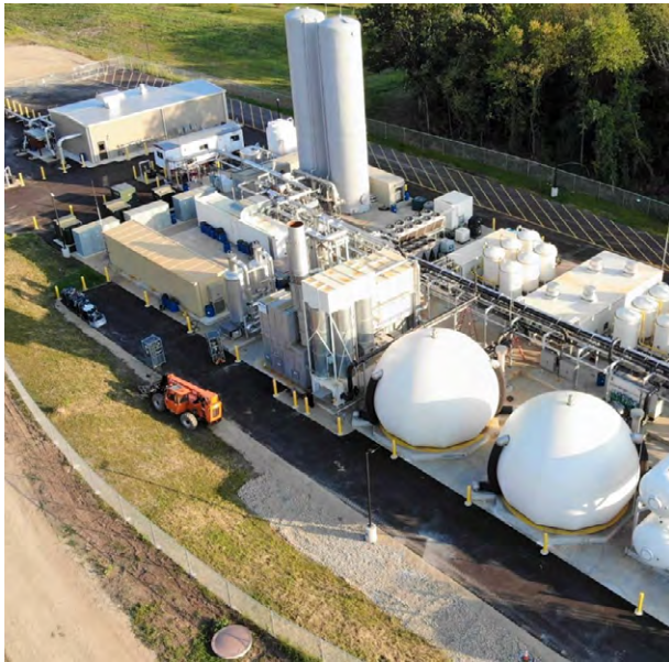
2-stage PSA landfill gas upgrading system
