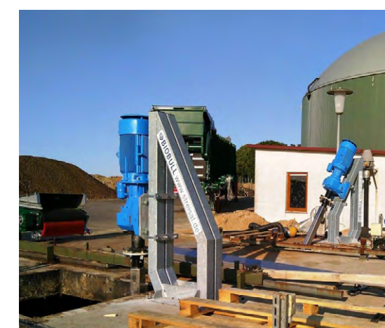
Hydrolysis tank with patented mixing system “streisal Hydrobull”
