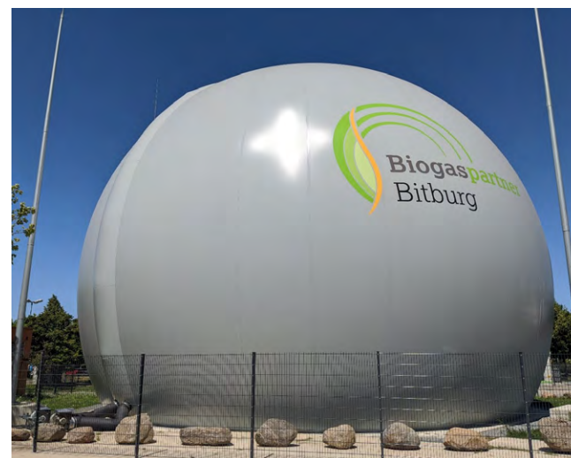
The low pressure double membrane biogas storage buffers 5.000 m 3 desulfurized biogas from 7 biogas plants.
