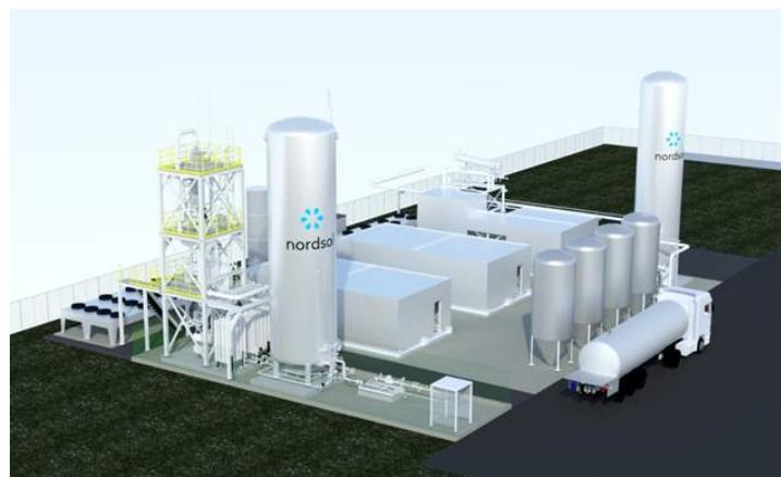
Nordsol is building the first bio-LNG installation in the Netherlands. The biogas for this installation is sourced from Renewi Organics, who produces biogas by processing organic waste. The iLNG technology from Nordsol upgrades and liquefies this biogas into bio-LNG. The offtaker of the bio-LNG is Shell, who sells it at LNG retail stations. The installation will produce 3,4 kton bio-LNG per year and 6,8 kton liquid bio-CO<sub>2</sub>.
